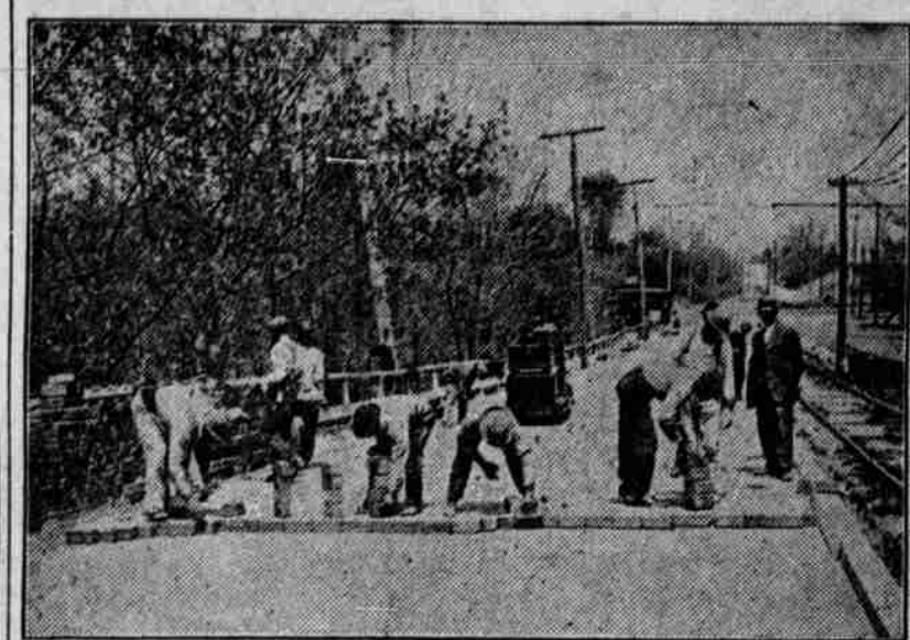
Laying Vitrified Brick for Country Road Pavement.
