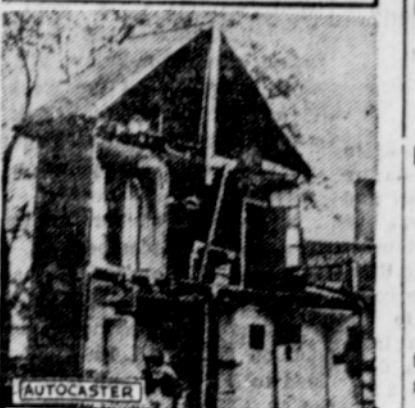
The owner of this slice of a house at East Milton, Mass., which was cut in half for the purpose of widening the street on which it stands, is fighting for damages against the town. The owner refused the offer for the property, but the town cut through anyway.
