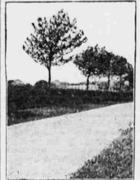
Well Kept Roadside Where Weeds Are Controlled by Frequent Mowing.
