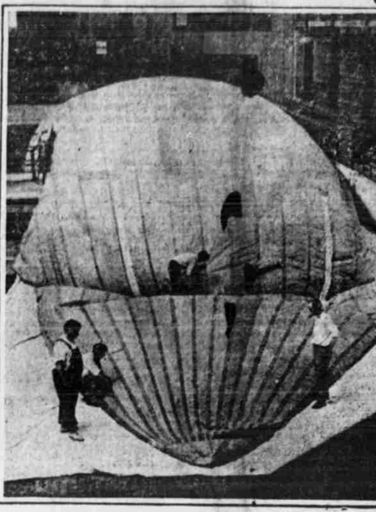
Photo by American Press Association. Many dirigibles are being built for our navy. Here is one being tested to detect flaws in the gas envelope.
