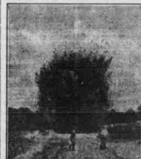
In loosening shale and rock to facilitate hand or steam shovel work dynamite is also very effective, while stumps may be blasted from the roadbed just as though they were being removed from a field to be cleared and cultivated.
