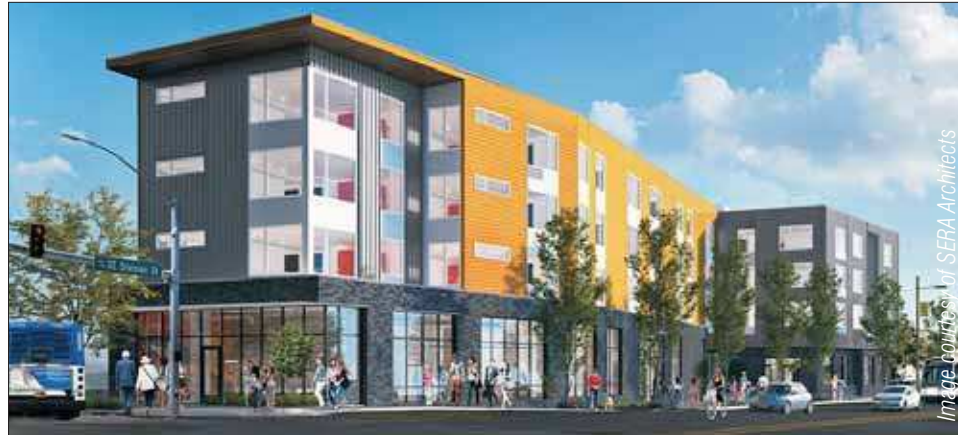
Photo courtesy of Metro
