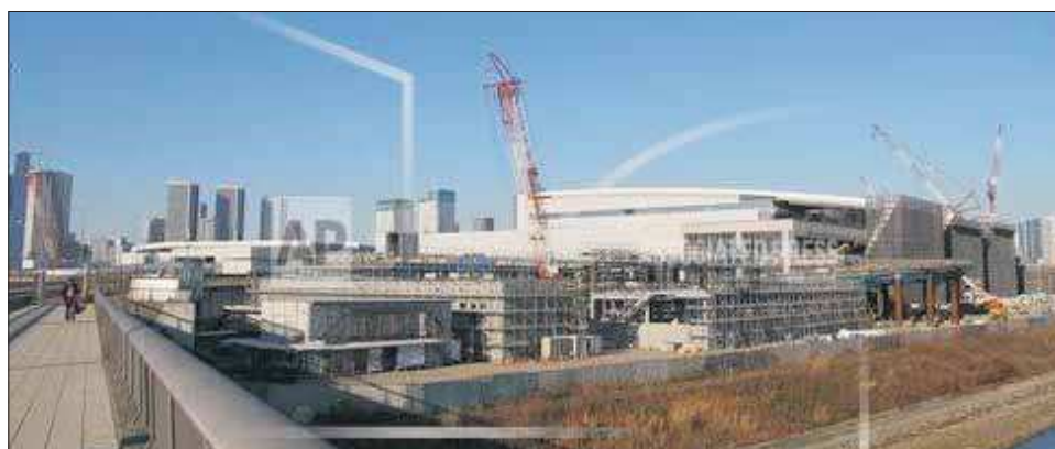
NETTING A NEW LOCATION. A man walks on a bridge by a construction site in Toyosu, in Tokyo, where a new market will open in 2016. In November, the 80-year-old Tsukiji market, the world’s biggest and most famous fish and seafood market, is due to move to the massive new complex further south in Tokyo Bay. (AP Photo/Elaine Kurtenbach)
