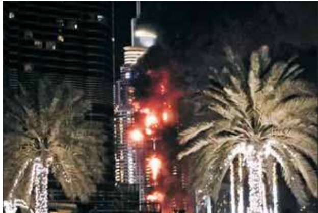
TOWERING INFERNO. A fire runs up some 20 stories of a building in Dubai, United Arab Emirates, on New Year's Eve. The fire broke out in a residential building near Dubai's massive fireworks display. (AP Photo/Jon Gambrell)
