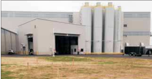
NORTH AMERICAN EXPANSION. Silos for holding carbon black, an ingredient mixed with rubber, oil, and other ingredients to make tires, stand next to the receiving area of the $300 million Yokohama tire plant in West Point, Mississippi. For Yokohama, the plant is its platform to fight for a slice of the competitive North American tire market. (AP Photo/Jeff Amy)
