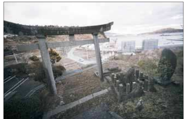
CEMENTING THE COASTLINE. A Shinto shrine gate remains standing on a hill while sea walls are built in the waterfront area of Rikuzentakata, Iwate prefecture, northeastern Japan. Four years after a towering tsunami ravaged much of Japan’s northeastern coast, efforts to fend off future disasters are focusing on a nearly 250-mile chain of cement sea walls, at places nearly five stories high. (AP Photo/Eugene Hoshiko)
