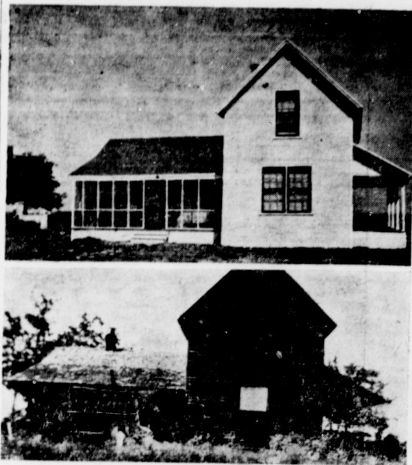
This transformation from old to new was worked largely by modern roofing and siding. Asphalt shingles provide a fire-resistant and colorful roof, which contrasts attractively with the new white sidewalls. One porch was screened in, windows were relocated, and a superfluous chimney was taken down. The dwelling is typical of many old structures that have sound, still useful framing.
