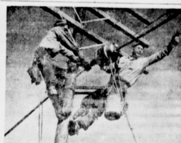
No one can guess the importance of the calls which will flow through the cable these linemen are installing.
