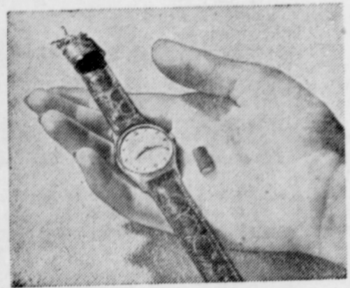
World's tiniest cell, a powerful energy capsule smaller than a penny in volume, provides power for new electronic watch.
