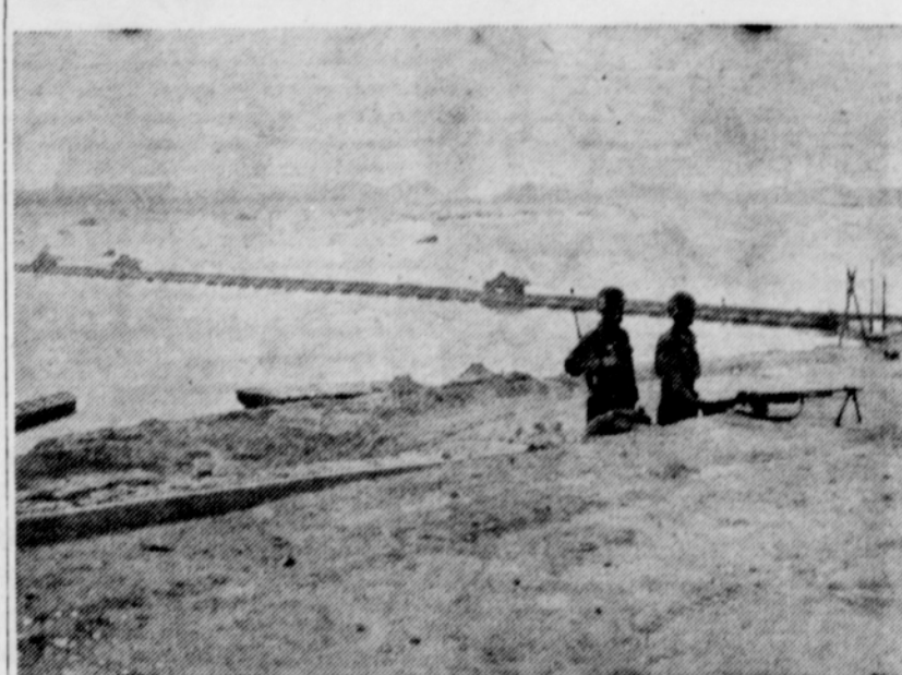
SUPPLY ROUTE ACROSS HAN . . . South Korean soldiers guard the northern end of the military pontoon bridge across the Han river as U.N. trucks shuttle between the north and south shores hauling supplies to U.N. forces holding a line north of Seoul. The Chinese Communist attempt to recapture the battered capital by May Day fizzled in the face of U.N. opposition here. Lt. Gen. James A. Van Fleet claimed a big victory.
