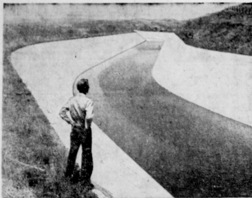
A general view of the Friant-Kern canal which carries central valley project water 153 miles from Friant dam near Fresno to the Kern river near Bakersfield. Concrete lining of the canal was completed recently, leaving only bridges and other structures to be finished before the full integrated operation of CVP begins in July. The canal has a capacity of 4,000 cubic feet of water per second.
