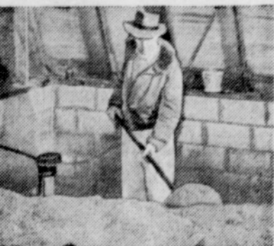
Brewers wet grains keep well in a tightly enclosed bin or store room. Unique feature of the store room on the Fritts farm is the pump (left hand corner) which constantly draws off excess water.
