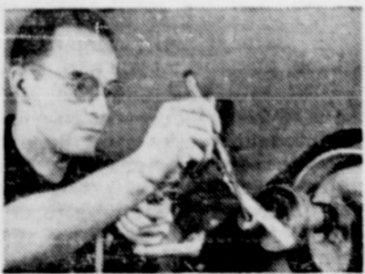
The end of a solid tube of glass is flared. This is the first step in making a tiny bubble tray used in a distillation column.
