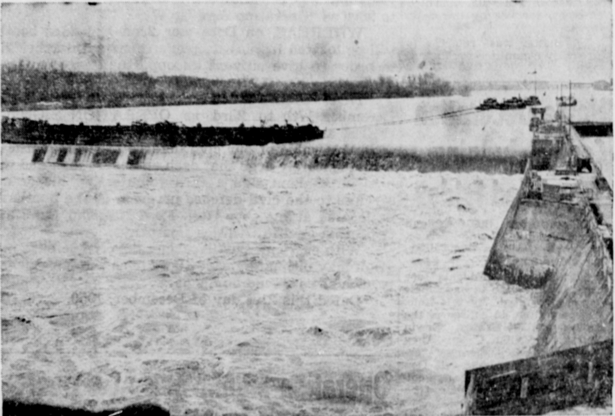
HAZARDOUS BUSINESS . . . A barge laden with gasoline clings stubbornly to the brink of the federal dam in the Hudson river at Troy, N.Y., as straining tugs finally pull it free. The huge barge, which was carrying 650,000 gallons of gasoline, lodged on the dam several days ago after breaking loose from a tug that was towing it in the strong and treacherous current of the rain-swollen river. Officials took every precaution to prevent a leakage of the gasoline upon the high waters because it might have created a fire hazard for several miles along the banks of the rampaging river.
