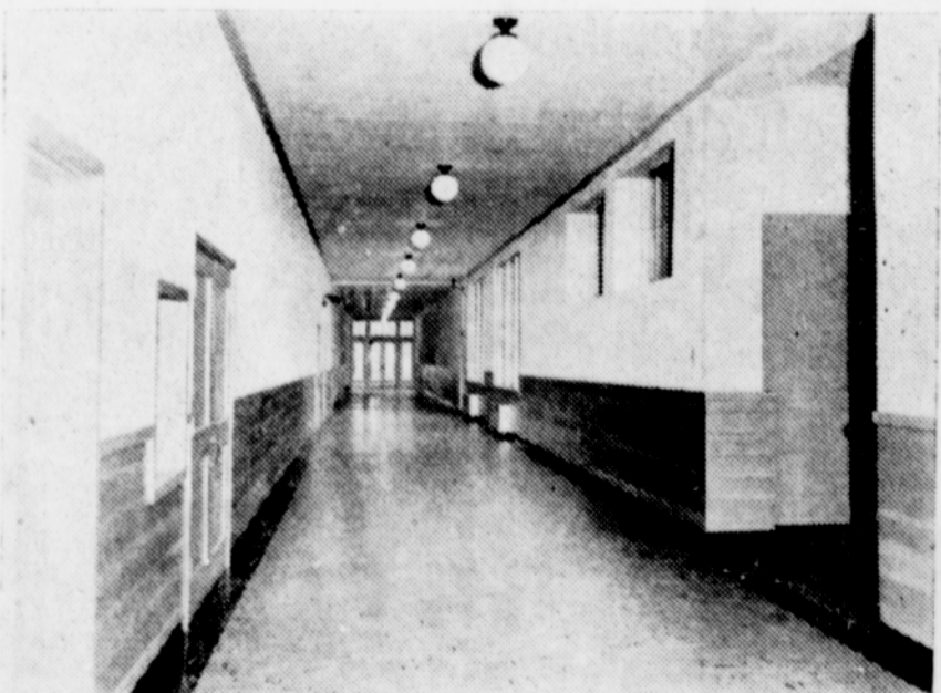
LIGHT, AIRY CORRIDOR —in Lincoln school is the latest word in school practicability. The wide corridor is easily kept spotlessly clean and designed to keep distracting noises at a minimum.
