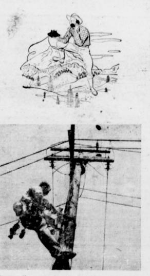
Power-line carrier is another new device which makes telephone communications possible in remote, sparsely settled districts. Your voice "hitch-hikes" dong existing power lines on radio waves that are tuned to follow the wires. Several power-line systems are now used on the Pacific Coast . . . and they're as safe and effective to use as any.
