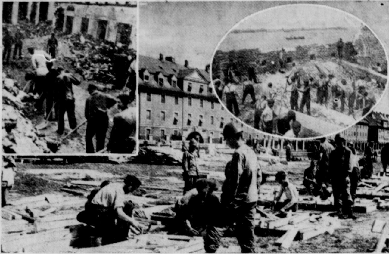
German prisoners, both war and civilian, are put to work as punishment for infraction of Allied military government regulations. They are forced to clean up wrecked buildings and to build beds for returning troops and civilians. At the Citadelle of Port Louis, Lorient, France, they uncovered mass graves of French civilians murdered by Nazis. Picture shows (inset, upper left): German prisoners cleaning up a street in Kitzinger, Germany. Oval: Uncovering a mass grave. Center: An assembly line at Munich making beds.
