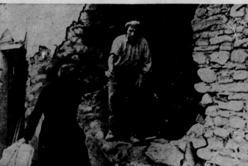
Even when it is in ruins like this one at Scarperia, near the Gothic line in Italy, there is no place like home. Using a shell hole in the wall for a door, the couple return and lay plans on building a new home without fear of further oppression from the Nazi yolk as was their lot in the past.
