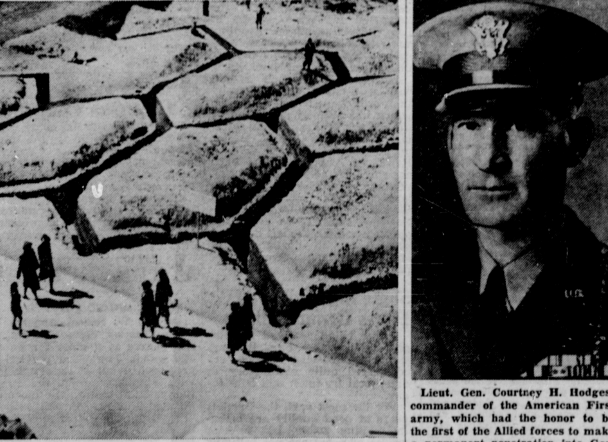
The slit trenches that cut up an area "some place in Italy" in a waffle-like pattern are being used by the Air WACs stationed near the headquarters of the 12th air force in Italy. This new type of trench is said to offer considerably more protection, and is harder to hit from air.
