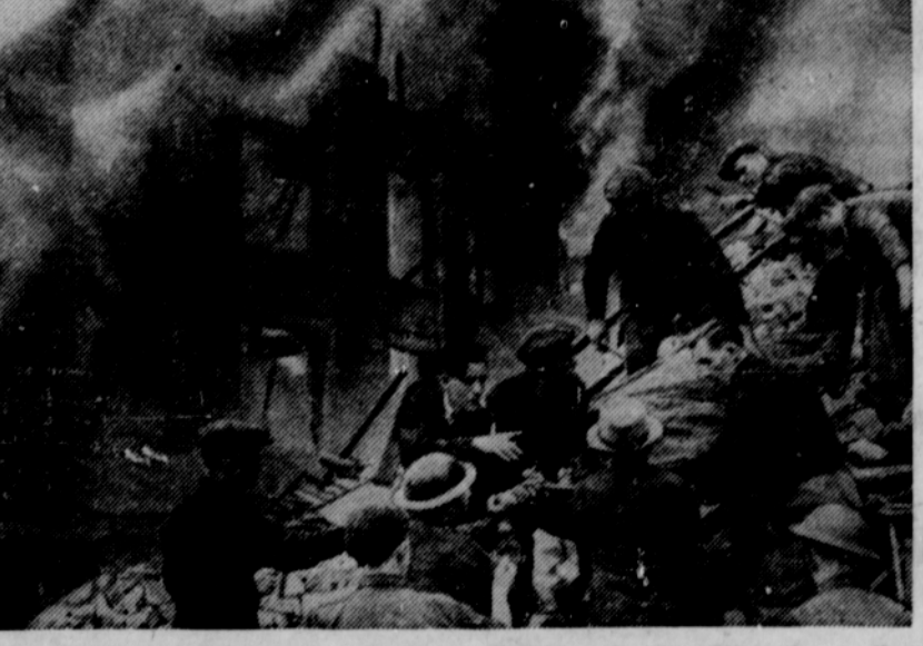
Air raid wardens and volunteers bring out casualties from the ruins of a block of flats struck by a German robot bomb in South England. Part of the building is still blazing in background. Recent figures released said that 17,000 homes are destroyed every 24 hours by the flying bombs. The total number of casualties caused by robots is not given.
