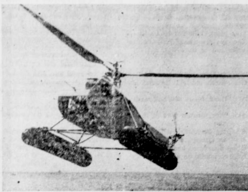
This type of helicopter, which will be built in quantity for the Army Air Forces by Nash-Kelvinator Corporation, peacetime manufacturer of automobiles and refrigerators, can alight on land, water, snow, thin ice, a rooftop or a parking lot. The craft can hover motionless in mid-air; descend and ascend vertically without forward motion and fly backward, sideways or forward with equal facility.
