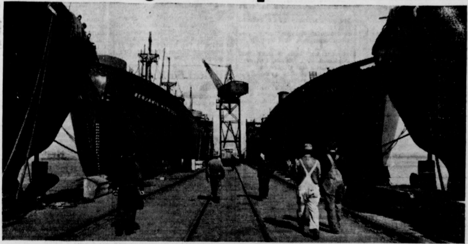
LIBERTY SHIP BEING FITTED OUT AT A BETHLEHEM YARD PREPARATORY TO SEA SERVICE. THE YARD IS PRODUCING A CONTINUOUS STREAM OF VESSELS OF THIS TYPE.
