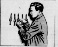
A regular check-up on pieces of X-ray film worn on workers' wrists helps guard against prolonged exposure to the rays given off by the X-ray tube.
