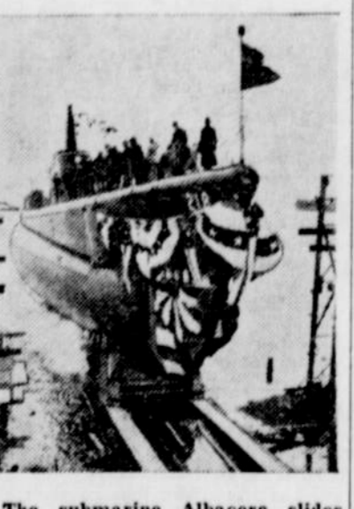
The submarine Albacore slides down the ways at yards of Electric Boat company, Groton, Conn. It was sponsored by the wife of Capt. E. F. Cutts, commander of sub base in New London, Conn.
