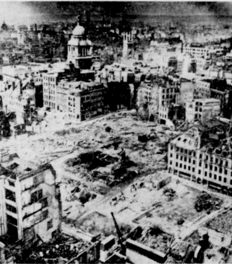
This photograph, just released by the British censor, shows some of the devastated sections in the great business center of London after air raid clearance work. An entire block of demolished buildings has been completely removed, leaving nothing but vacant lots, as shown in the picture. Hardly a building escaped damage.
