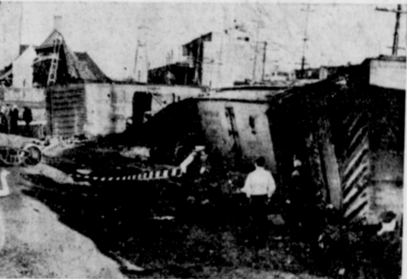
The Grand Trunk & Western railway's passenger depot at Lansing, Mich., was wrecked when a freight train jumped the track and crashed into it, killing one person and injuring several. Photo shows general view of wrecked train and depot. It is believed a wheel on a freight car broke. The train was traveling 60 miles per hour.
