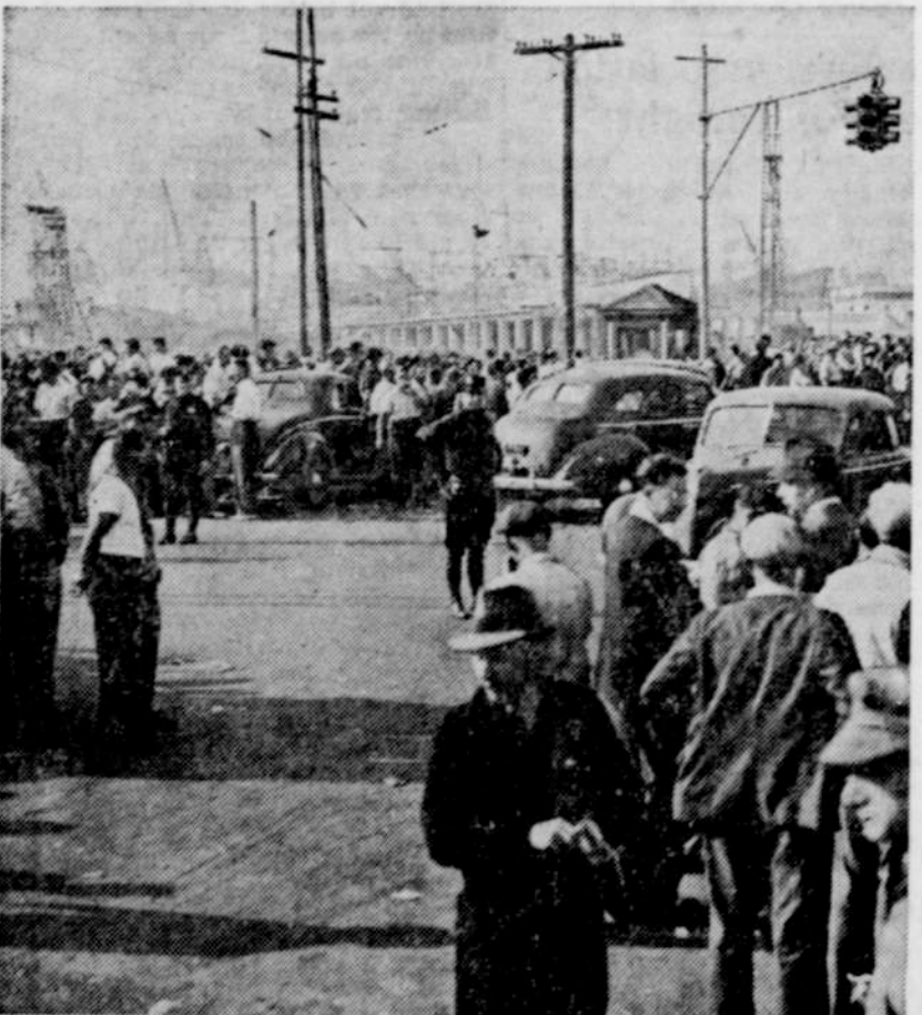
While work on some $373,000,000 worth of warships and merchantmen remained at a standstill, these members of the C.I.O. industrial union of America picketed outside the yards of the Federal Shipbuilding & Dry Dock company at Kearney, N. J. The strike was called over the failure of the company and the union to agree in a dispute over the classification of some 1,500 workers.
