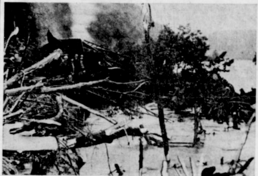
Roaring waters of the Youghioghenny river, sent far over its banks by a three-day continuous rain, washed out the tracks of the P. & L. E. railroad and sent this freight train plunging into the river at Dickerson Run, about 30 miles from Pittsburgh. The three-man crew was riding in the engine cab and narrowly escaped death.
