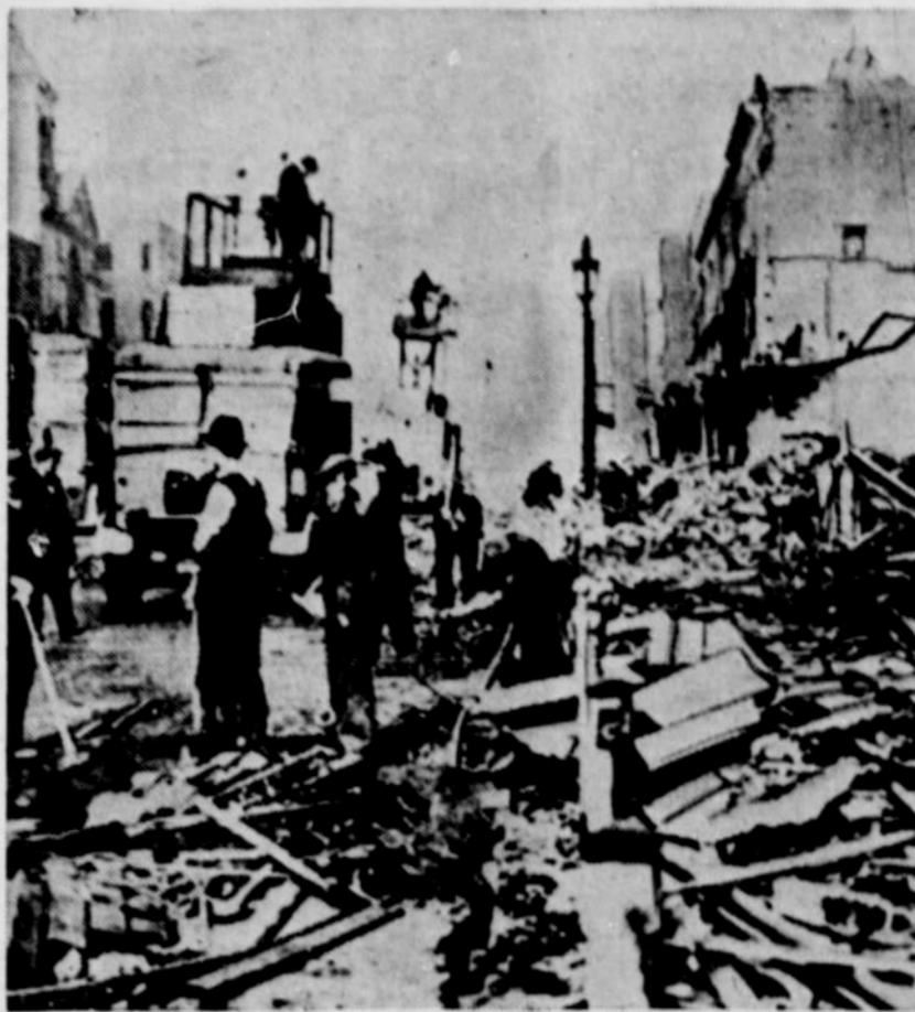
After what is believed to be the worst air raid of the entire war on the capital of the British empire, workers are shown clearing up the debris in London, while the work of digging the dead and wounded out of the ruins was still going on. Material damage was terrific, thousands of high explosive and incendiary bombs having been dropped.
