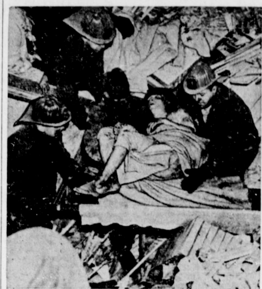
Members of four families in Cincinnati, Ohio, were blasted out of their beds by a pre-dawn explosion that wrecked a three-story downtown tenement building, and killed 13 members of five families. A dozen others living on upper floors were injured. Photo shows firemen removing injured victim from the scene of the explosion.
