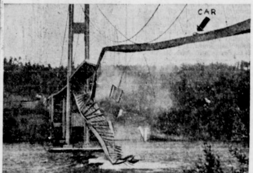
This soundphoto shows the new Narrows bridge at Tacoma, Wash., third longest single suspension span in the world, as it started to disintegrate and fall 190 feet into Puget Sound. The bridge was completed last July at a cost of $6,400,000. Note the car on the bridge which was abandoned by its occupants as the bridge began to collapse.
