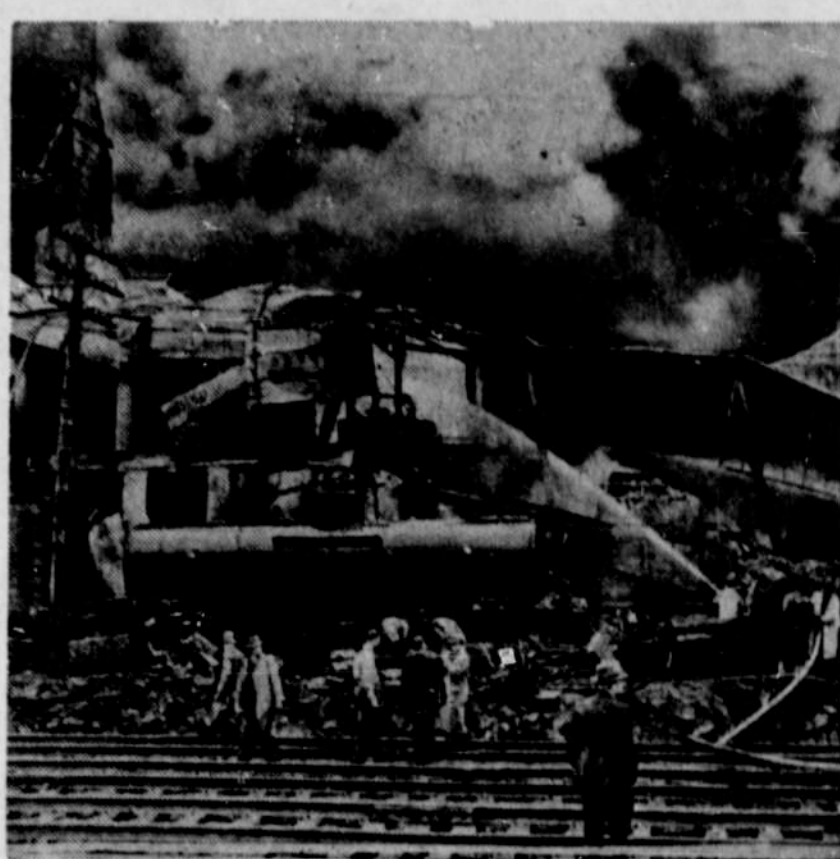
The burning ruins of two buildings are shown in the above photo of the Pennsylvania Industrial Chemical corporation at Clairton, Pa., which was damaged by an explosion of resin and oils. The blast resulted from "adverse chemical reaction" in an agitator. Six persons were injured in the blast. The damage is estimated at $50,000. Flames were brought under control an hour after the explosion.
