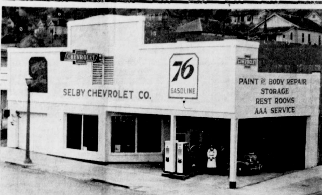
THE newly remodeled and redecorated front of the Selby Chevrolet company, above is shown as Lloyd Selby prepared for his formal opening from 3 o'clock to 6 o'clock tomorrow afternoon, April 15, at which time visitors will be shown this city's latest business improvement which includes not only the front modernization but also streamlining of showroom, offices, service, lubrication and paint and body departments. Shown in the picture are Verne Hastings, car sales; Frank Culp, service manager, and Selby, standing beside a 1939 Chevrolet sedan. New computing pumps, included in the improvements, are shown in the new drive-in entrance. (Bushnell photo.)
