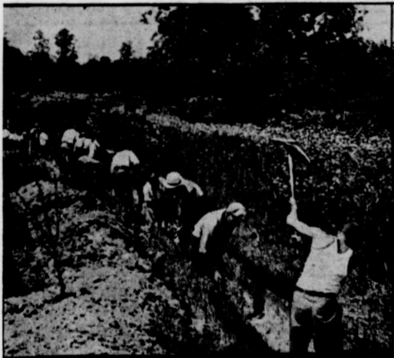
Workers are shown digging a water-line ditch, as work started on the housing project at Heightstown, N. J., where 200 subsistence homes are being erected on a 1,270 acre plot by the Federal Housing administration.
