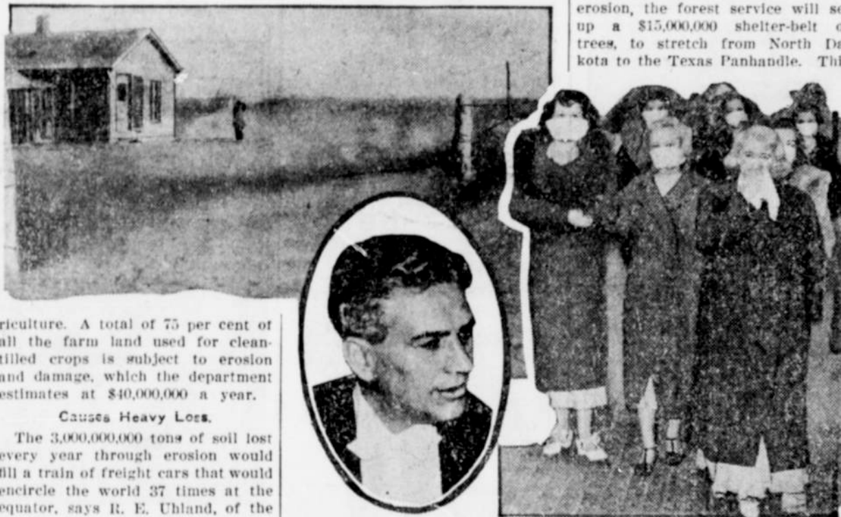
Top, Ranch in Colorado Piled High With Dust. Below, Left, Dr. Rexford Tugwell, in Charge of Erosion Control. Right, City Folks Also Have Their Battle With Dust.
