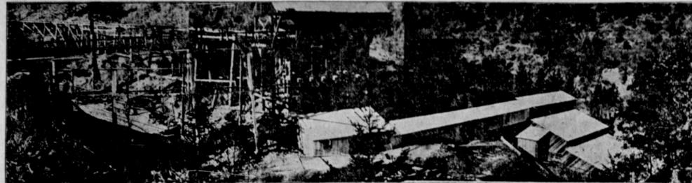
The lowest tunnel portal of the Pacific States gold mine one and one-half miles west of town is on a level with the huge upper ore bin shown in this picture. The bin towers above the 100ton daily capacity flotation gold mill which is built on the mountain slope in approved fashion.
