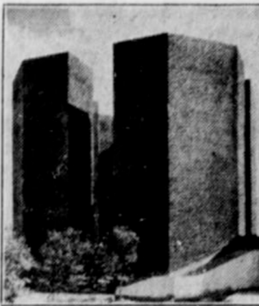
These are cypress trees, whether you like to be told that or not. Of course they are something of a modern conception, but they are still architectural cypress trees. They are in a court in the Electrical group of the new 1934 Chicago World's Fair, which opens June 1
