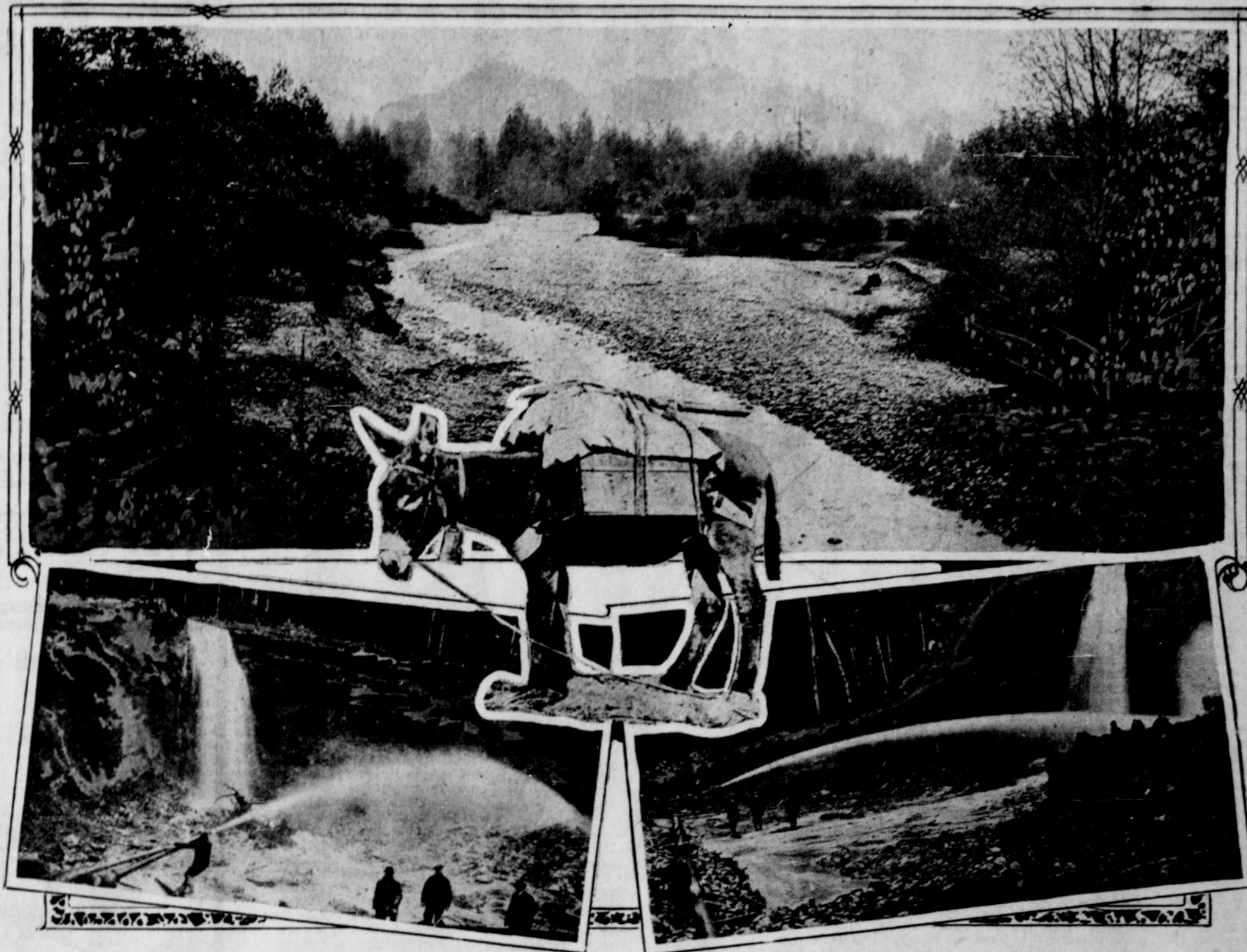
GOING AFTER GOLD IN APPLGATE—Top photo shows Little Applegate channel from which placer gold has been mined. Bottom views show giants working on 40-foot embankments at Sterling mine on Little Applegate. Inset shows a miner's hay-burning motive equipment.
