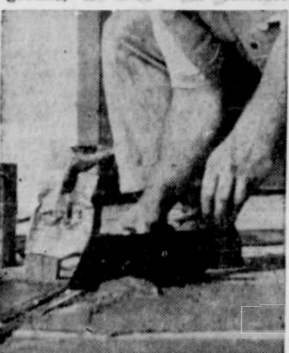
Greased form, set on levelled ground, is filled with concrete.
