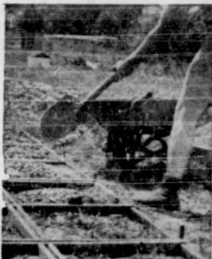
Greased form, set on levelled ground, is filled with concrete.
