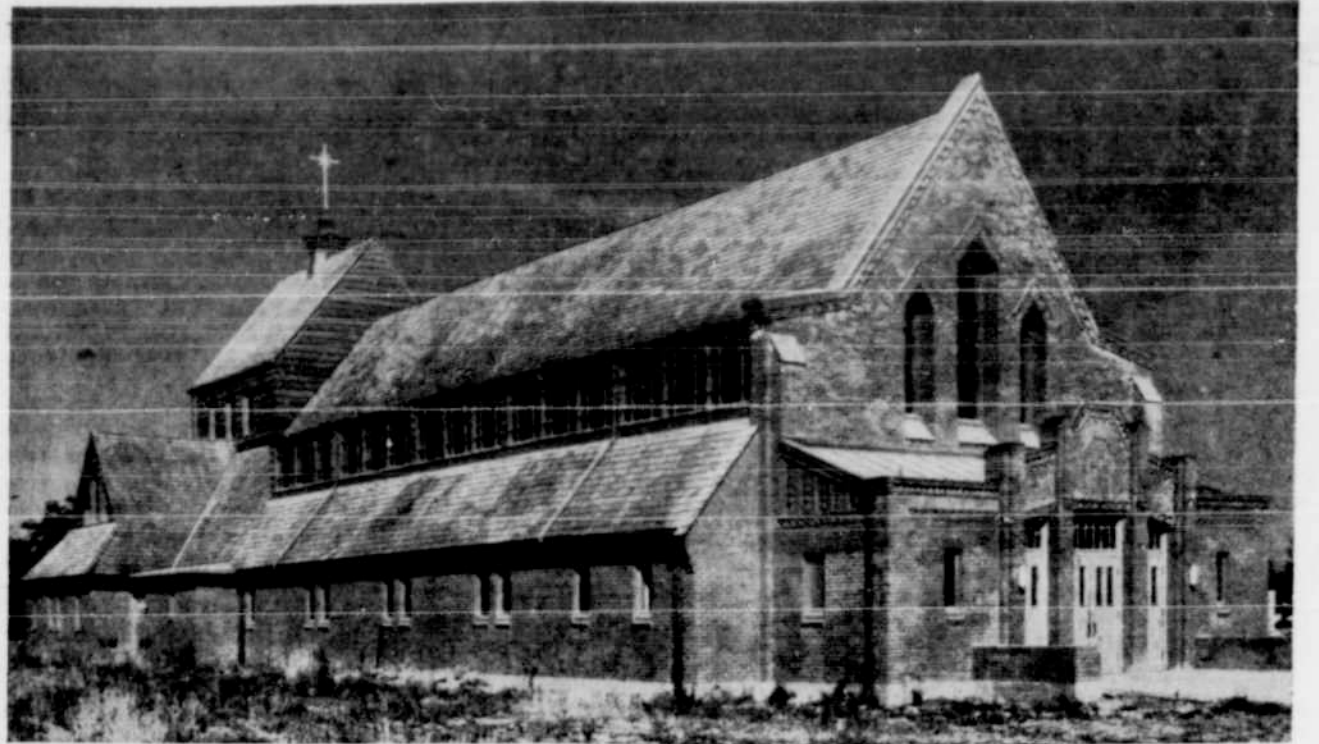
Erected on the corner of Fifth and Franklin, on land donated by Father George O'Keefe, St. Cecilia's new church is the first of three buildings to be completed. The parish hopes to erect a parochial school and rectory on the four acre site, soon. (Photo by Harrell - Beaverton 4988)
