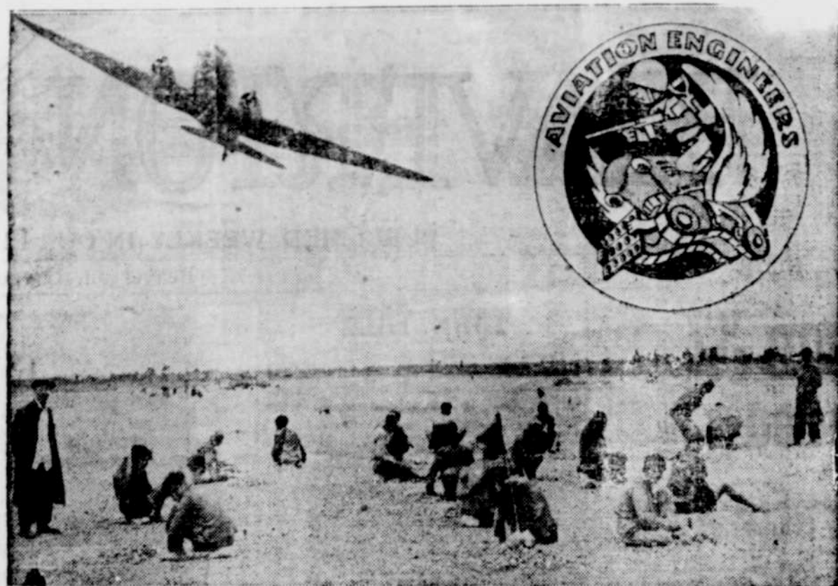
Released by U. S. War Department, Bureau of Public Relations AAF AIR FIELD IN CHINA —Willing Chinese labor, working under methods of 1,000 years ago nevertheless soon convert a tilled field into a first class runway for the 14th American Air Force. Uncle Sam's tireless Aviation Engineers direct the job. Inset, "bucking bulldozer", unofficial insignia of the Aviation Engineers. (Army Air Forces photo).
