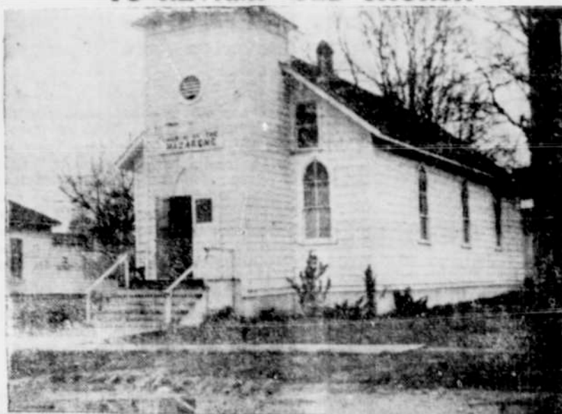
One of Beaverton's oldest structures, the Nazarene church, is being reconstructed.
