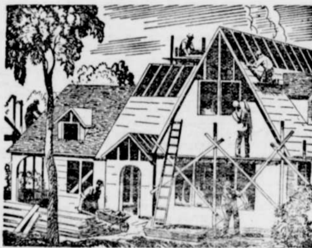
Photograph of one of the many modern homes now under construction in the Tualatin Valley.
