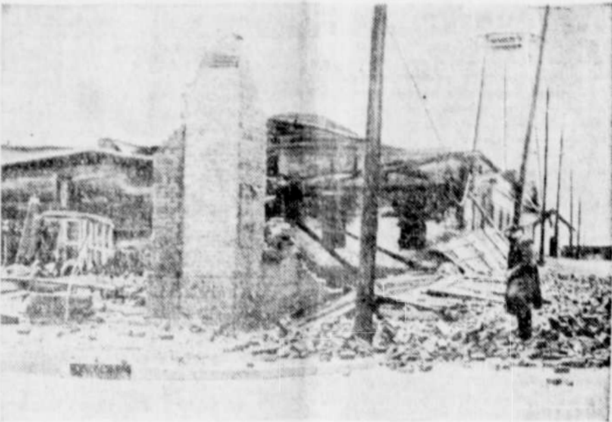
The Watkins building at Jackson, Ga., wrecked by the recent wind which assumed cyclopic force and wrought heavy property damage.
