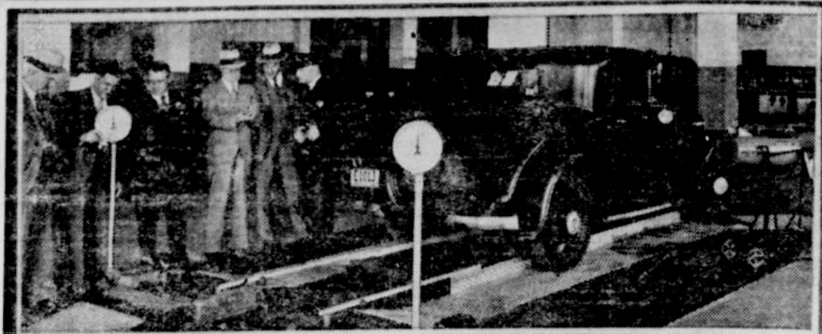
National Safety clinic inspection machine manufactured by Bendix Products corporation which was installed last week by Thompson & Dubey. First use of the device was witnessed by city traffic officials, motor club officers and the press, with a police car being the customer. The device checks all safety factors.
