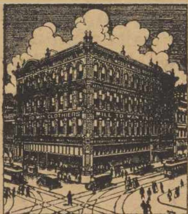
WOOLEN MILL BUILDING
